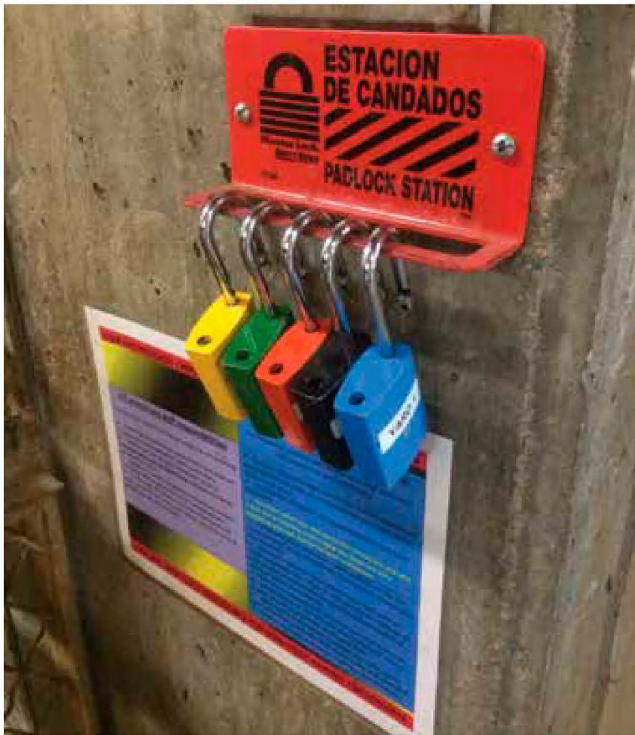
Example of an engineered control: “Lock Out Tag Out” system.
