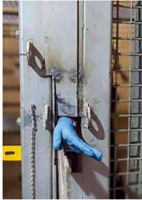
Shift door between two holding areas that had an opening while the door was in the open position where an animal could reach through. When the door was closed, the gap was not there.
