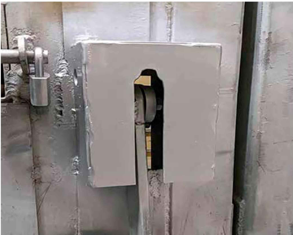
To prevent the hand-sized gap that appeared when the shift door was open, a welding contractor created this box that allows the keepers full use of the door; including opening, closing, and securing it. Pictures taken by Ann Marie Felhofer.
