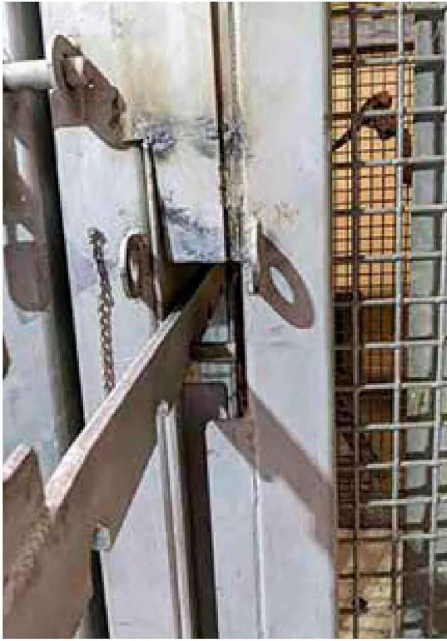
Shift door between two holding areas that had an opening while the door was in the open position where an animal could reach through. When the door was closed, the gap was not there.
