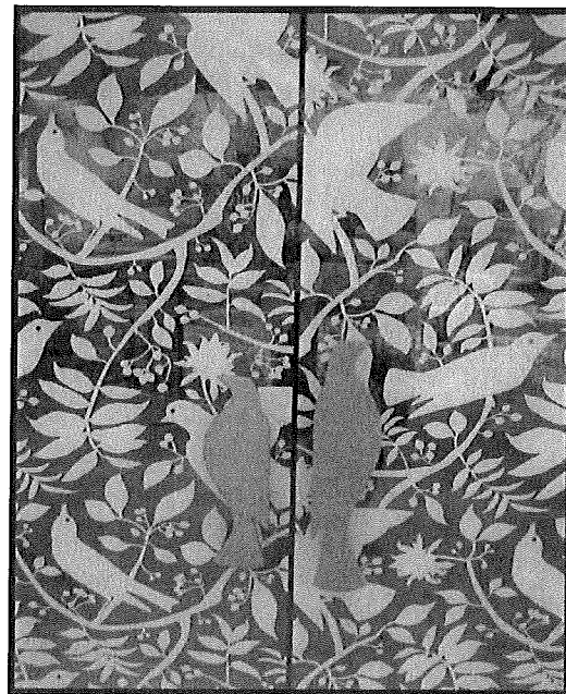
Bird-friendly entry doors to the McNeil Avian Center at the Philadelphia Zoo
